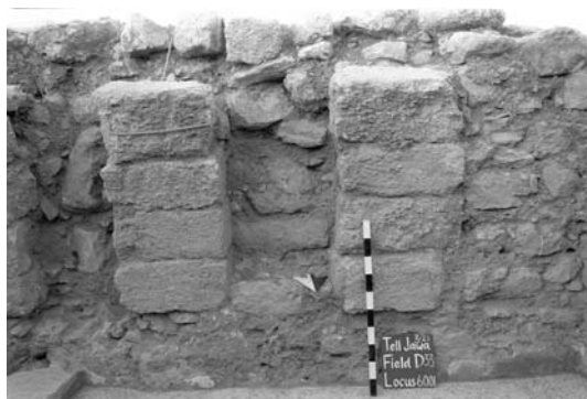
Figure 3.21. Arch D33:19 (left) and 20 (right) built into south Wall 6001.
